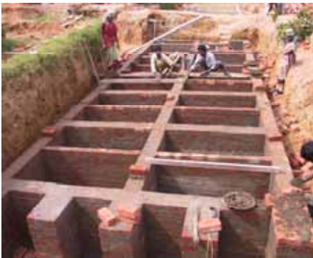
Technical layout of a DEWATS unit in Mekarsari Jaya, Indonesia (right) – constructed, good integrated DEWATS plant on a field (above) – Anaerobic unit of the DEWATS system under construction (left)
